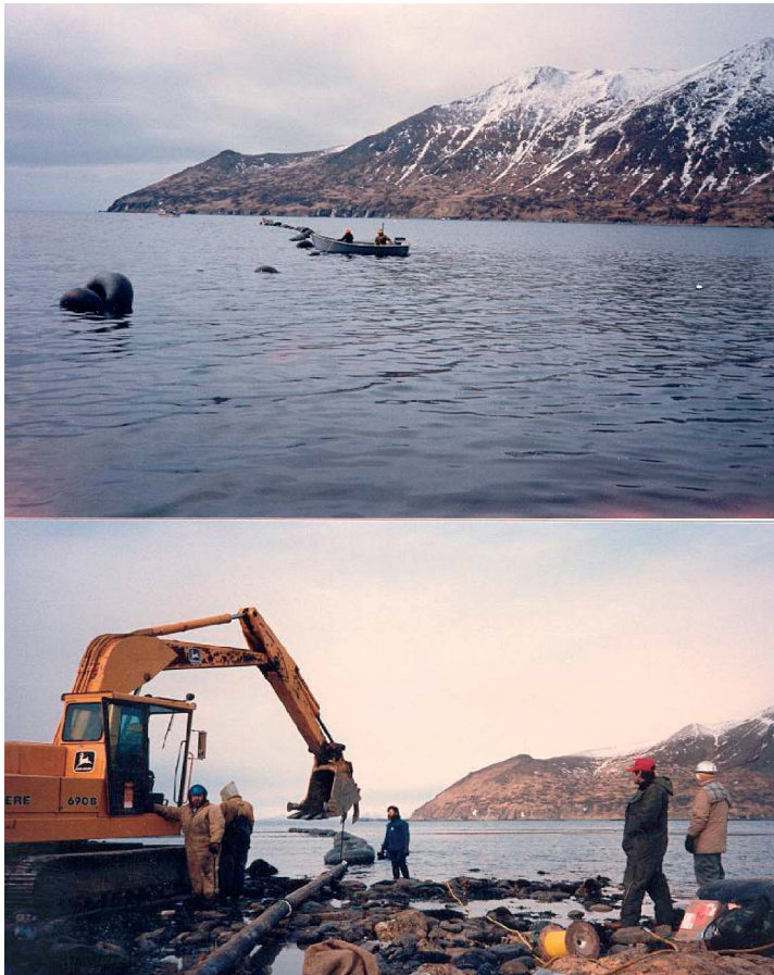
Figure 7.5 Installation of a ductile iron submarine outfall in Alaska by flotation and submergence
