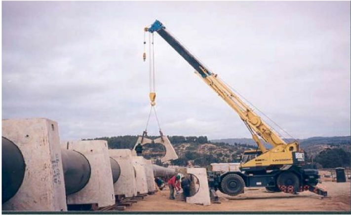
Figure 10.9 Mounting concrete ballasts on the Loma Larga outfall, Valparaiso, Chile (courtesy Belfi-Montec)
