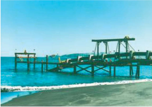
Figure 10.20 Temporary launching trestle for HDPE pipe
