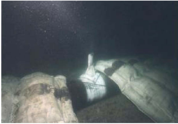
Figure 9.11 Concrete block mattress for stabilization of an outfall diffuser (Courtesy Ivo Van Bastelaere, PEng)
