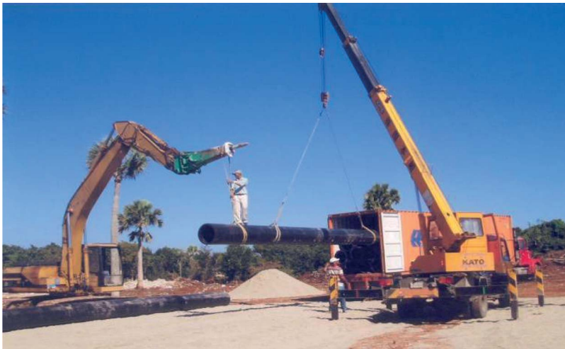
Figure 10.2 Unloading HDPE pipe from a container using nylon straps to protect the pipe from abrasion
