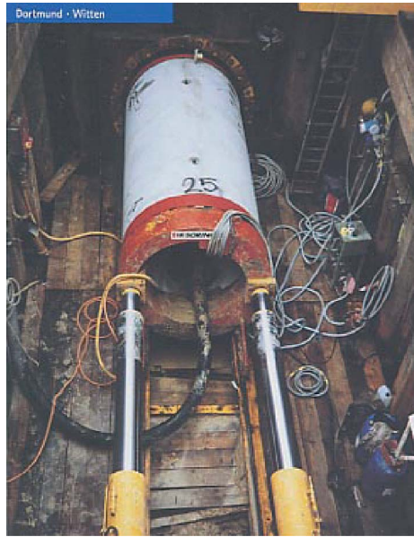
Figure 11.9 Concrete pipes being jacked in behind a TBM (Courtesy of Herrenknecht AG)
