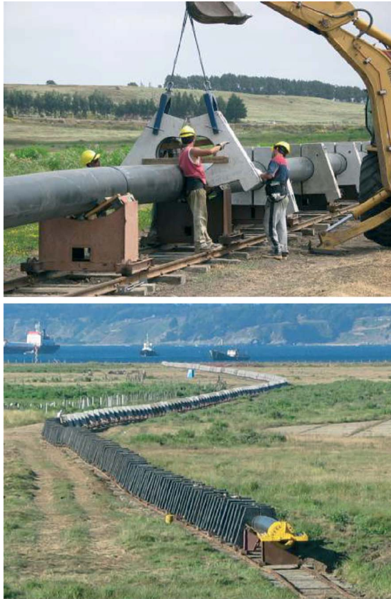
Figure 10.4 Temporary rail system used in constructing the outfall for Quintero, Chile (courtesy of Belfi-Montec)
