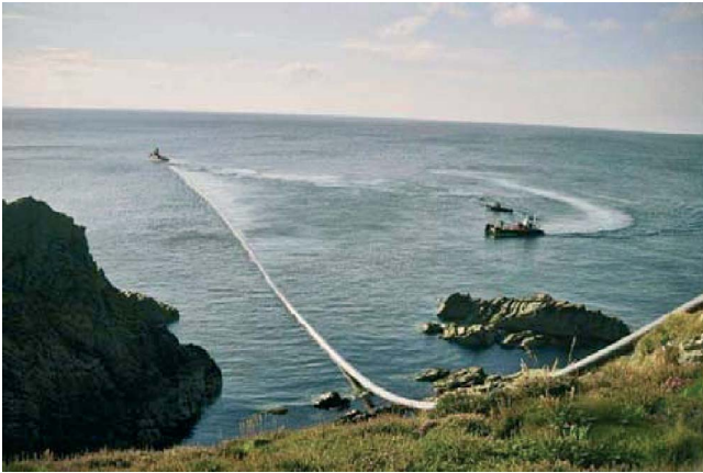
Figure 11.23 Towing the HDPE pipe out to sea (LMR Drilling)
