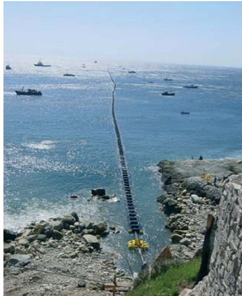
Figure 10.13 Floating and positioning an outfall for submersion in Quintero, Chile
