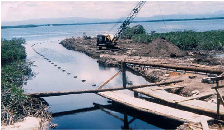
Figure 10.10 Locally constructed gantry used for launching a small diameter submarine pipeline 3,800 m long for Placencia, Belize
