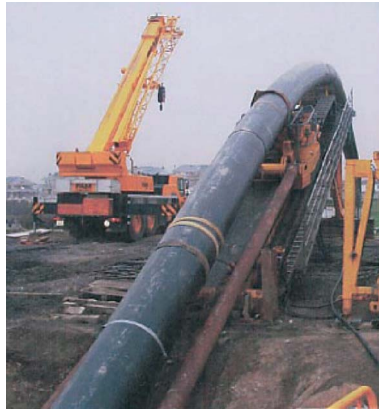
Figure 11.21 Pullback of 900 mm diameter HDPE pipe (Haustadt & Timmermann)
