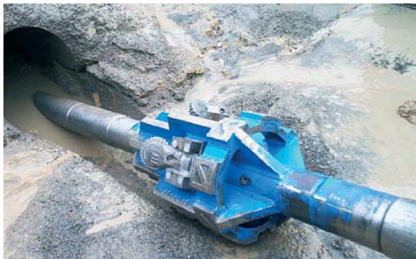
Figure 11.22 Hole opener assembly (LMR Drilling)
