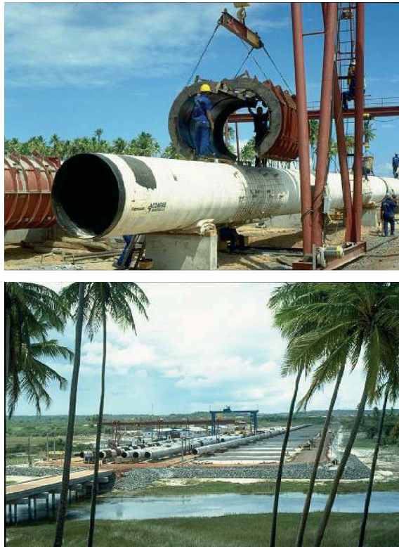
Figure 10.17 Steel outfall 1.34 m diameter, 4,800 m long to be installed by bottom pull in Salvador, Brazil
