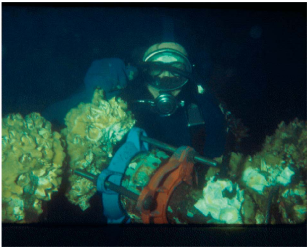
Figure 8.7 Heavy growths of marine organisms on a submarine pipeline 8 years after installation in Angoon, Alaska (Reiff)
