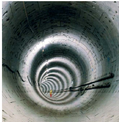
Figure 11.5 Segment lined tunnel
